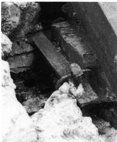
Fig. 15 North end of tie-bar in chancel east wall
