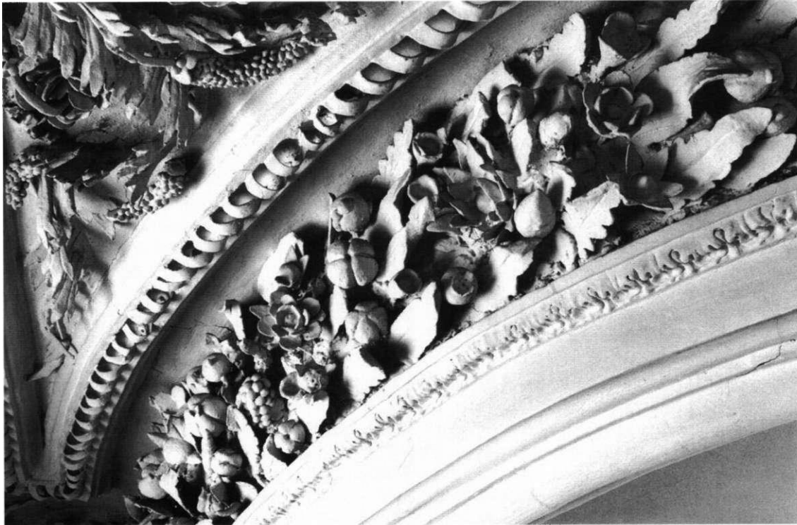
Fig. 1 Detail of nave ceiling
