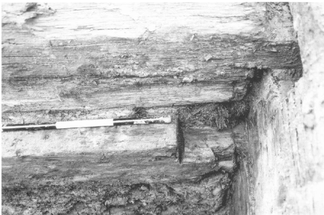
Plate 7 Joints between F113/F153 and F130/F135 from the south
