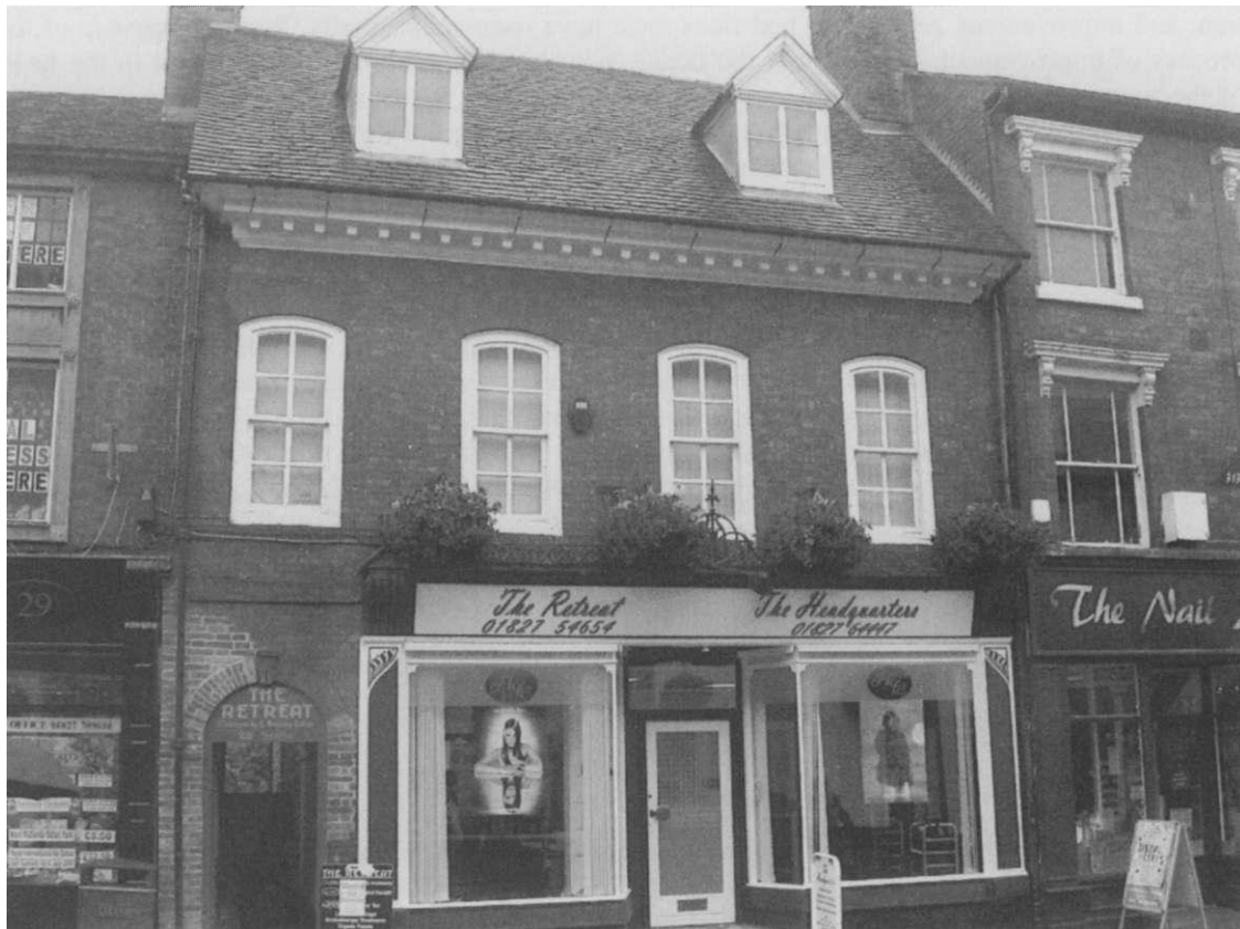
Fig. 2 No. 30 Market Street: the house of 'Mr Meacham', built c. 1726 (Photograph: M. Kingman).
