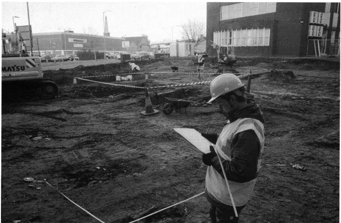
Plate 2 The site during excavation, facing north
