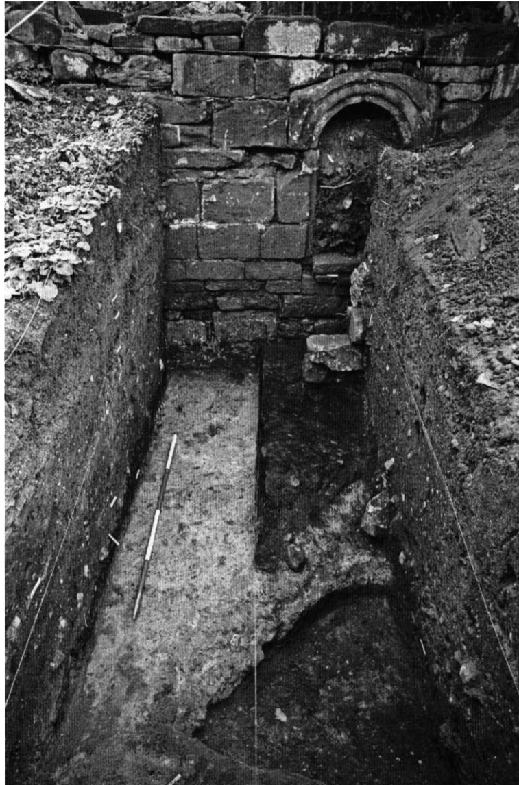
Plate 1 The masons' working floor (1027) from the north
