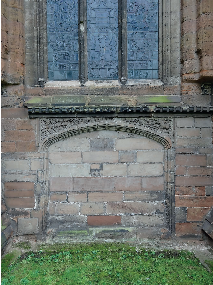
Fig. 5 The entrance to the chantry chapel of Dean John Yotton (d. 1512) located adjacent to the tomb of St Chad in the second bay of the nave. (Photo © author)
