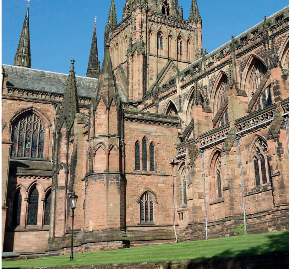
Fig. 3 Exterior of St Chad's Head Chapel, Lichfield cathedral. (Photo © Lichfield Cathedral Photographers)
