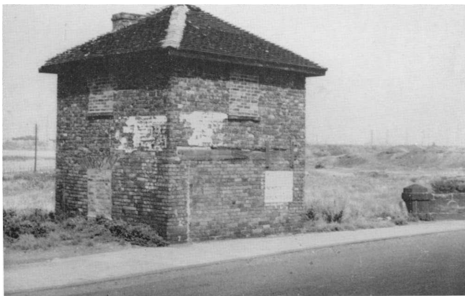
Plate 1b Toll House, James Bridge, Darlaston (Staffordshire), 1960
